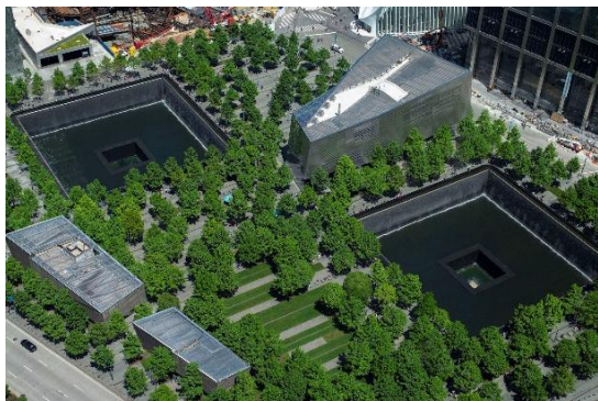
(a) Memorial pools created within the footprints of the Twin Towers (Lee, n.d.)
